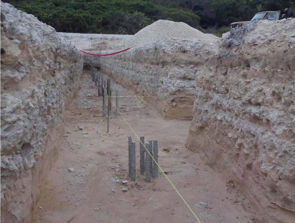
Picture 5: Pile installation complete
