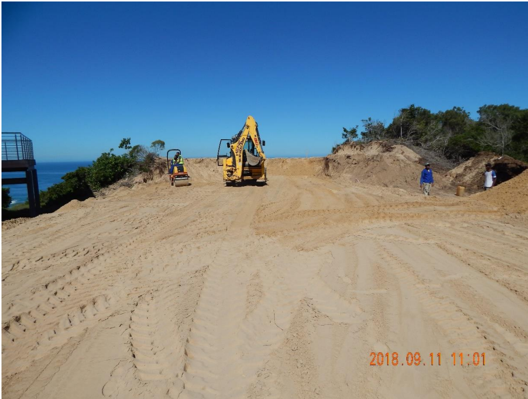
Picture 2: Site levelled and preparing for G5 material to be imported
