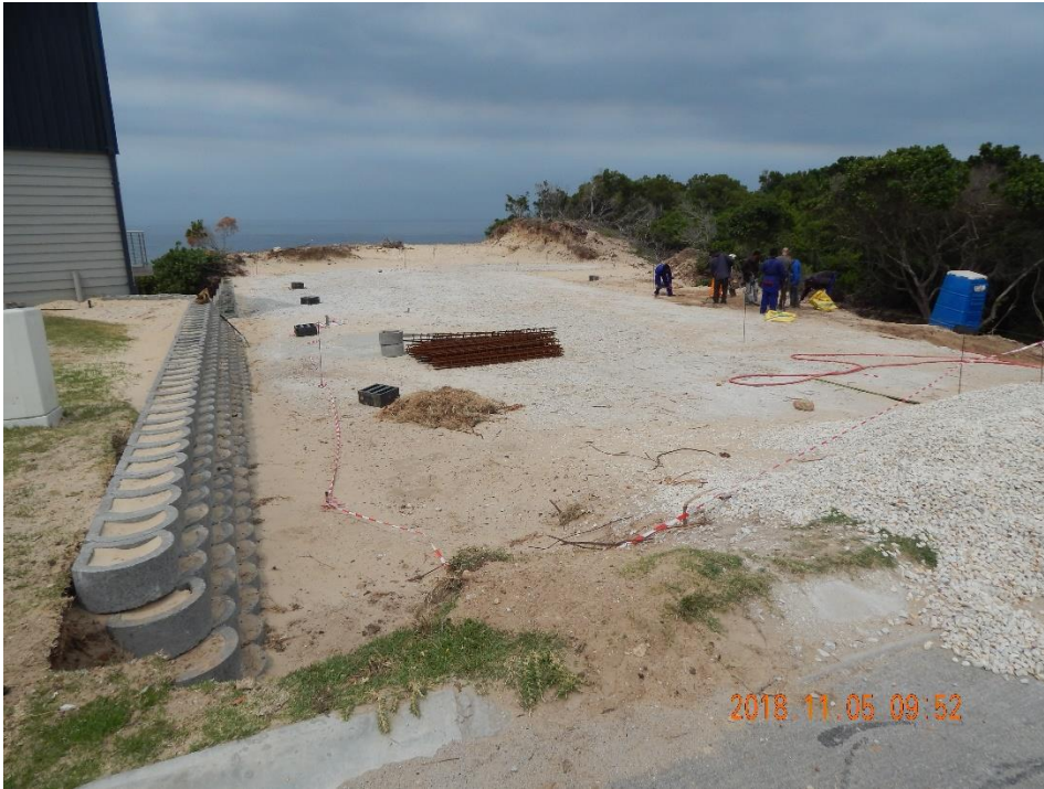
Picture 3: G5 material imported for platform
