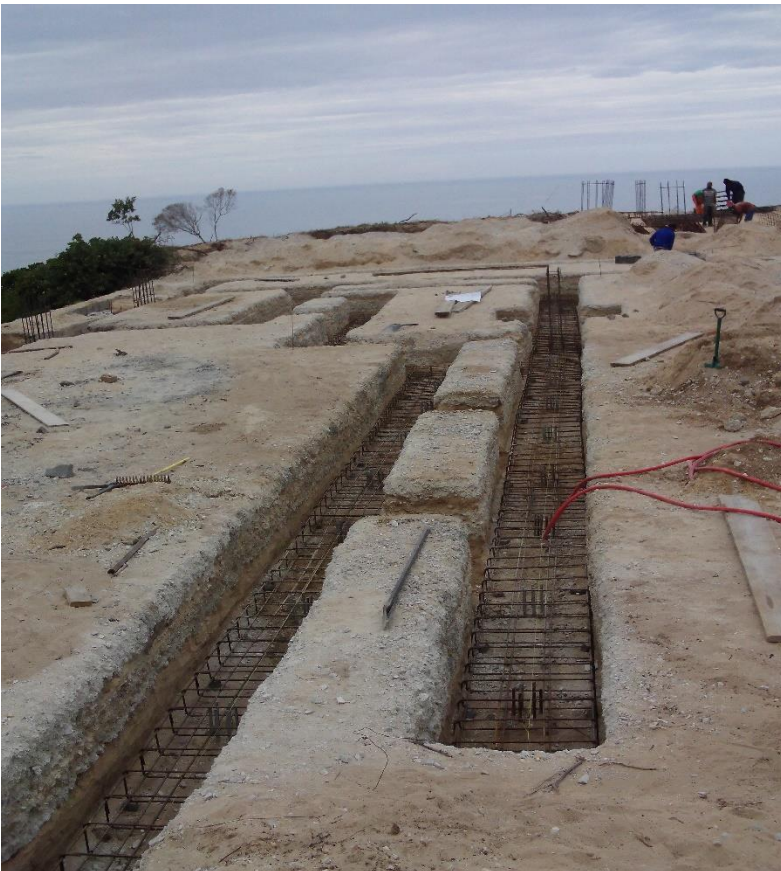
Picture 6: Foundation reinforcing installed
