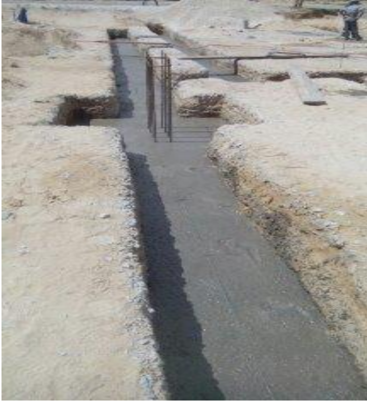
Picture 6 : Foundation concrete poured
