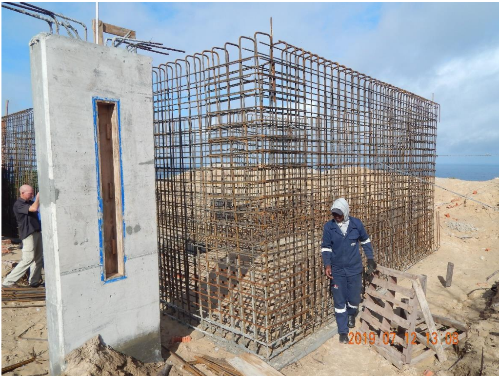
Picture 7 : Pool wall reinforcement being installed
